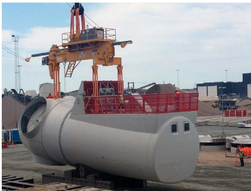
Here we see the 360 tonne 'nacelle' being prepared for lift.
